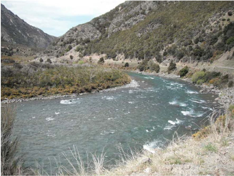
Hurunui River looking across at the proposed tunnel intake for the FGL Scheme.
